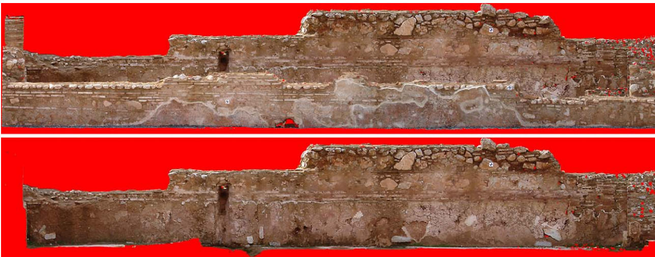
Figure 14. Orthoimages of part 2 from 17 images (top). Below is the projection of the posterior wall from the same images.
