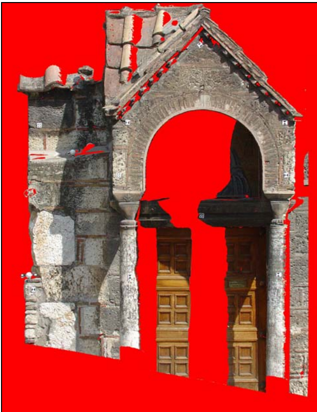
Figure 4. Orthoprojection (below) of the image above. At the right silhouettes of the columns texturing problems are seen.
