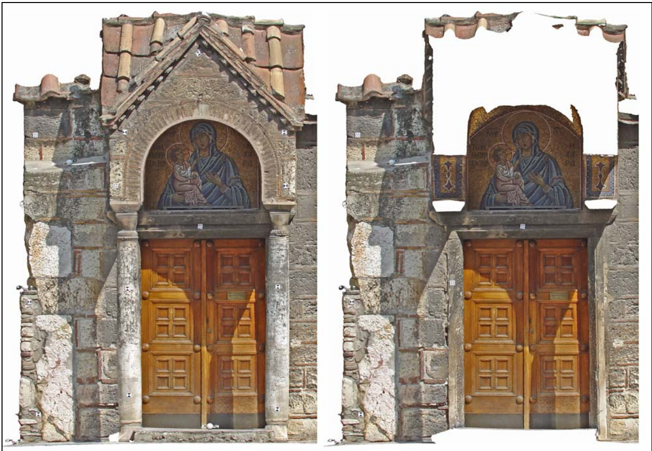
Figure 6. Left: Extract of the orthoimage from 7 images. Right: orthoprojection of a model section defined by a maximum Z-value.
