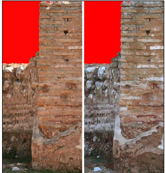
Figure 11. Orthoimage details of part 1 generated by blending texture from 8 images of two different images sets.
