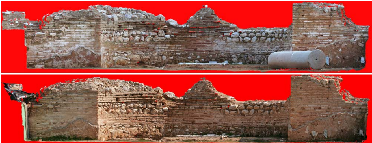
Figure 13. Orthoimages of part 1 from the two image sets (top: 16 images, bottom: 23 images).
