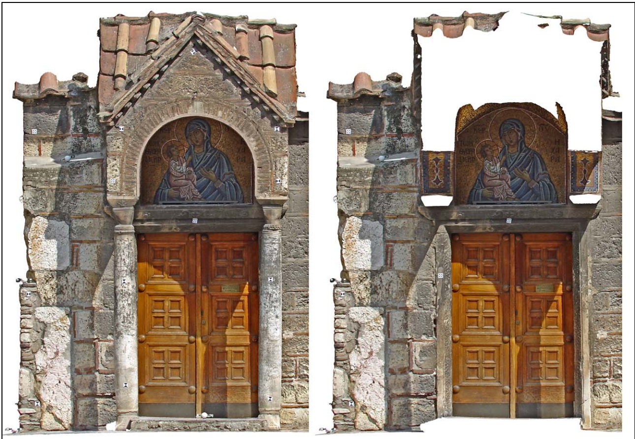
Figure 8. Left: Extract of the orthoimage from 7 images. Right: orthoprojection of a model section defined by a maximum Z-value.
