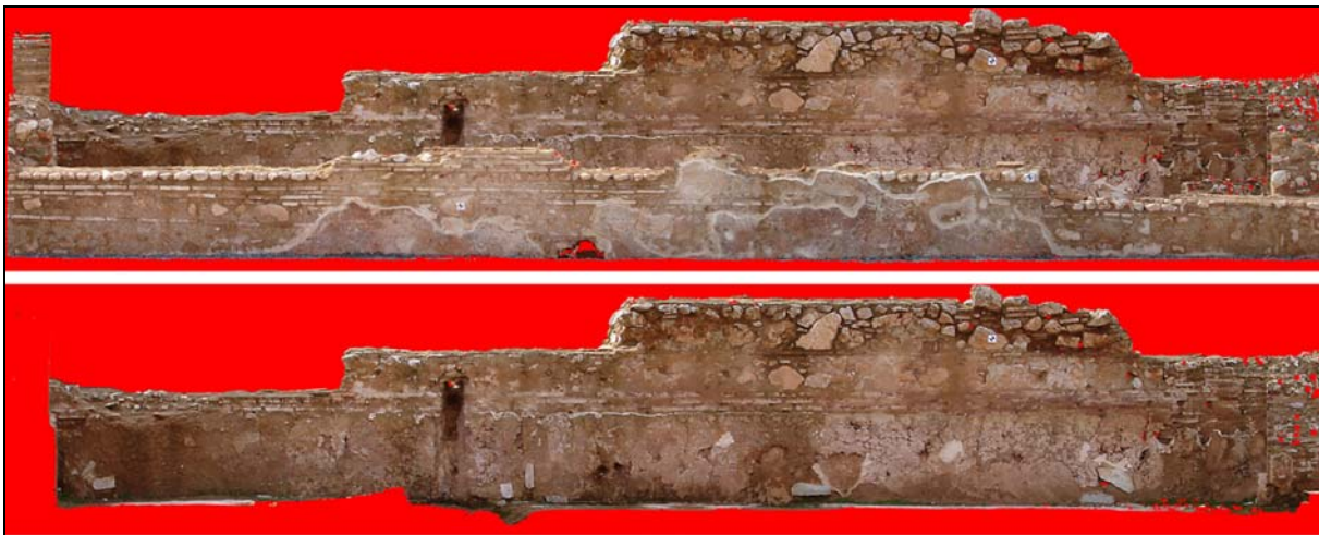
Figure 13. Orthoimages of part III from 17 images (top). Below is the projection of the posterior wall from the same images.
